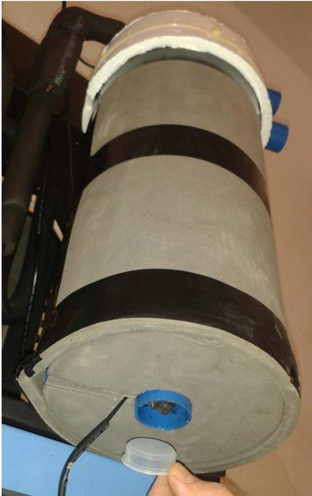
*Remove the rubber cap positioned in the chiller's bottom side.*
